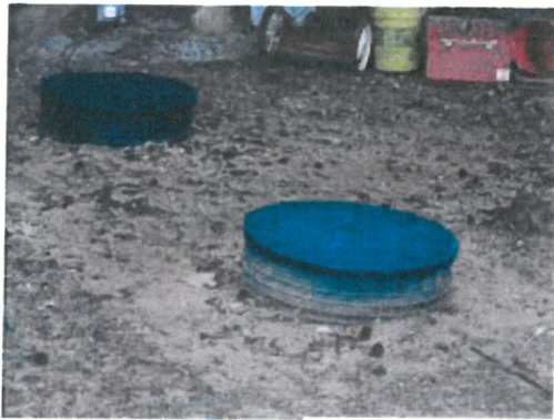
New Risers on Existing Tank
