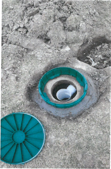
New baffles & risers installed on an existing tank (both inlet & outlet shown)
