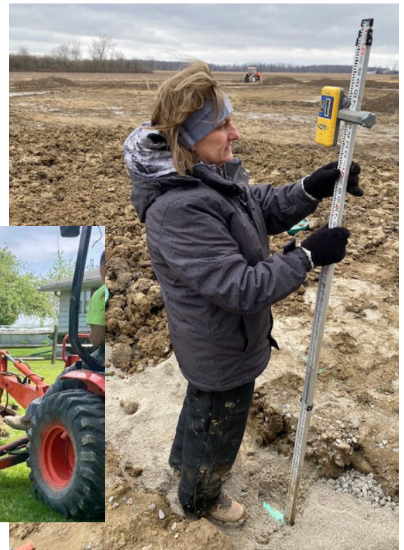
Sheila D'Aguanno, REHS, checking the fall in the line from the house to the septic tank. Sewage system contractor replacing a distribution box for a leach field.
