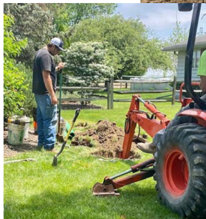
Sheila D'Aguanno, REHS, checking the fall in the line from the house to the septic tank. Sewage system contractor replacing a distribution box for a leach field.
